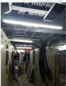
INSTALASI KABEL FIDEER
