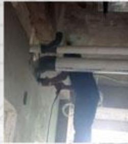
INSTALASI PIPA AIR KOTOR
