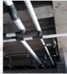
INSTALASI PIPA AIR KOTOR
